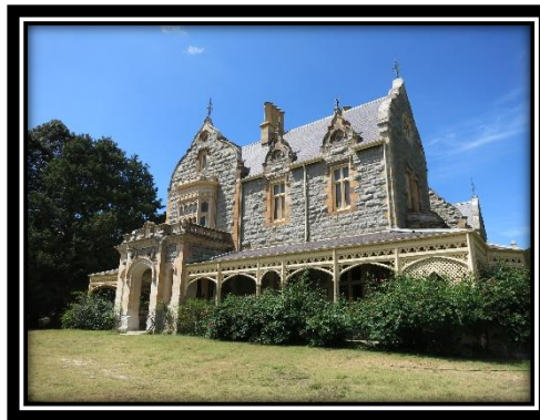
Fig 21. Abercrombie House constructed substantially from local granodiorite (photo: Chris Marshall).
